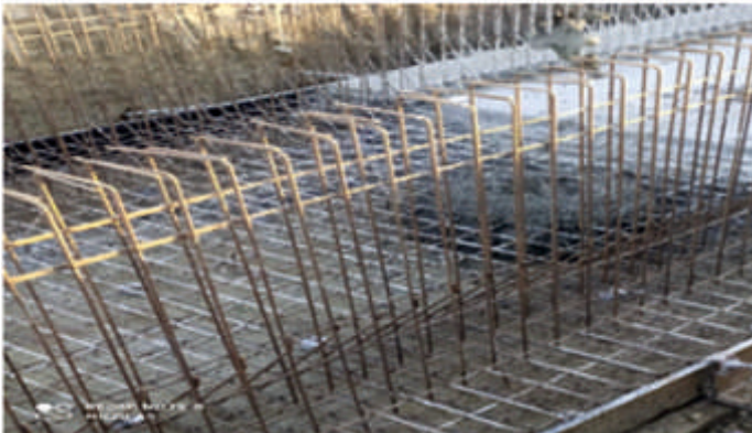
RCC work at Drain in progress
