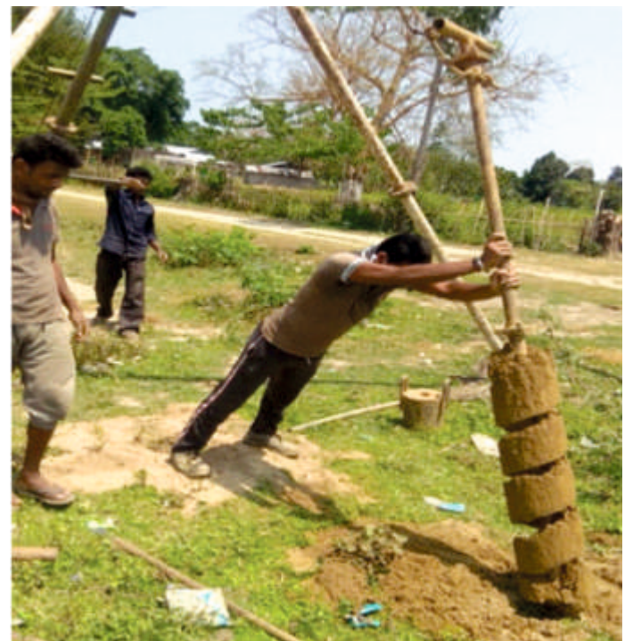
Soil exploration work completed
