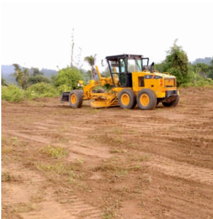
Site Cleaning Work in Progress
