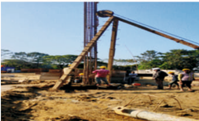
Reinforcement casing lowering at ATC site
